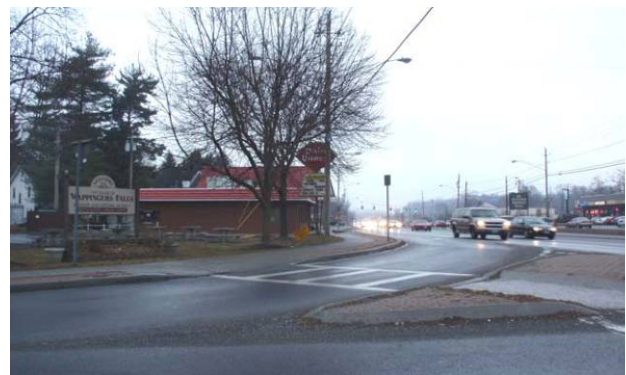
Figure 14 - Existing Route 9/East Main Street intersection
